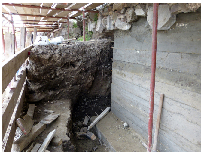
Figure 7. Sozopol – process of hypothetical restoration with concrete of a medieval fortress (NINCN archives)
