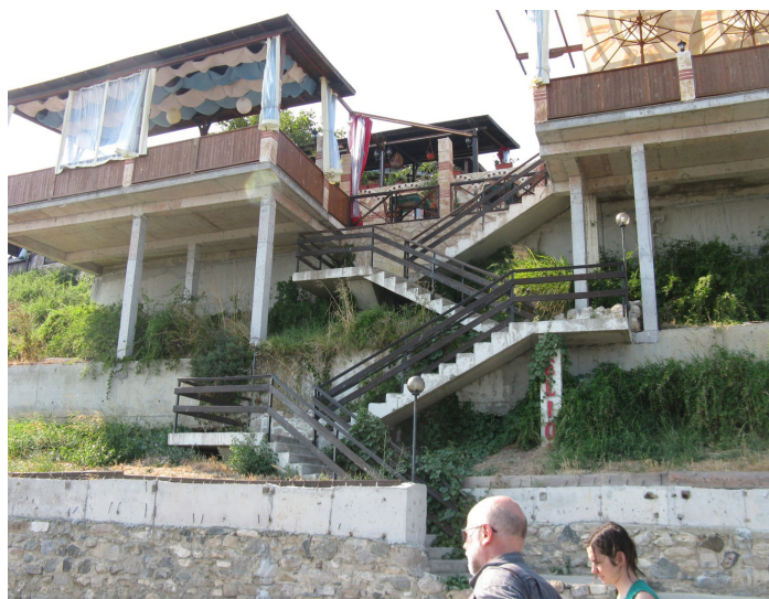
Figure 3. Illegal construction in Old Town of Nessebar (2011)
