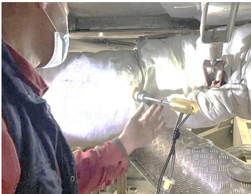
Figure 5. Installation of exhaust sampling probe
