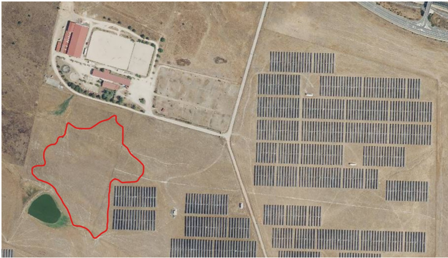
(a) Solar panels
